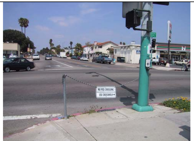
A chain barrier like this would be sufficiently detectable to blind pedestrians if there was also a lower chain, attached so that at its lowest point, it was a minimum of 6" from the walking surface.
