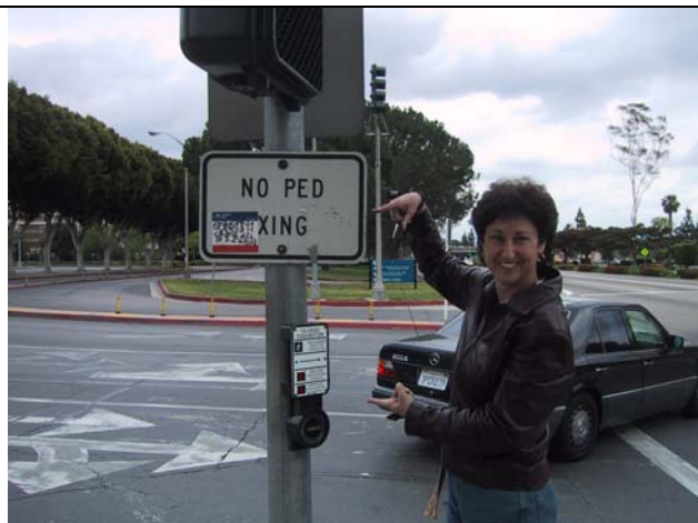
The only crossing permitted from this corner, which has an accessible pedestrian signal, is a diagonal crossing from the apex of the corner. Although the tactile arrow is correctly aligned, most pedestrians who are blind would assume that the arrow was simply oriented incorrectly.
